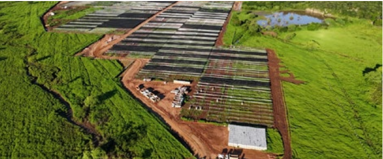
Mauriti PV DOBT Project, Brazil
