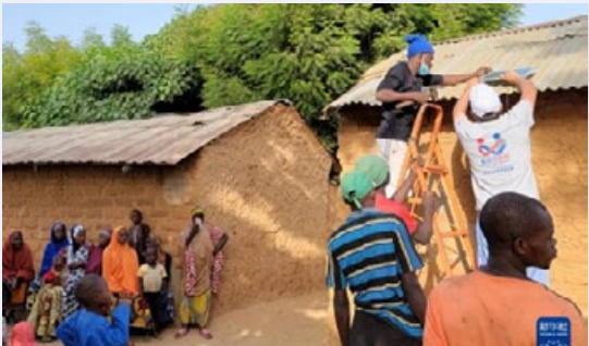
Installation of Solar Lights
