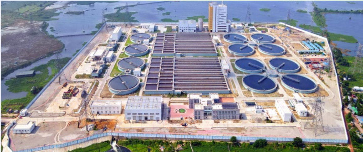
Dasherbandi Sewage Treatment Plant in Bangladesh
