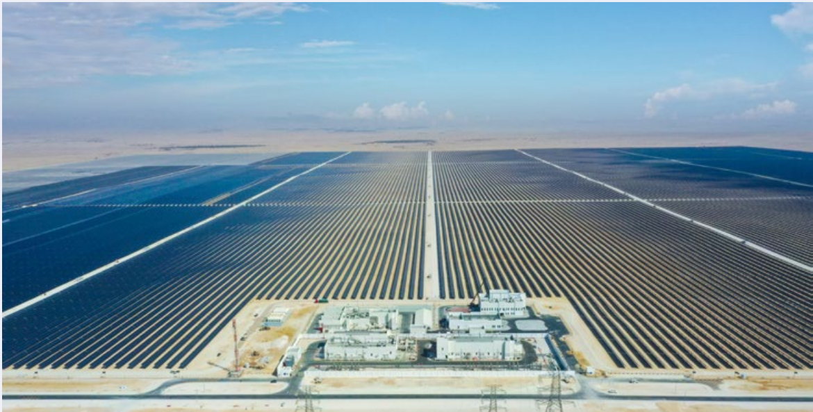
Qatar Al Kharsaah Solar Power Station
