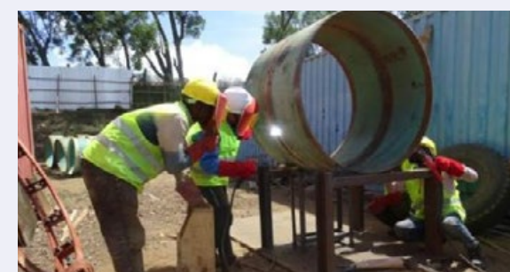
Steel Tube Welding Training
