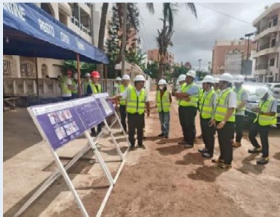
Work on site by inspection team
